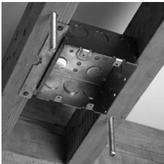
4" junction box and 8" bolt circle Figure A
