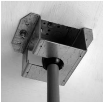
Hang straight bracket and pendant Figure B
