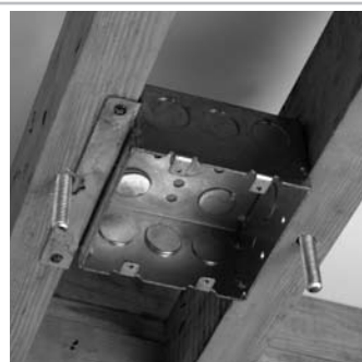
4" junction box and 5-3/4" bolt circle Figure A
