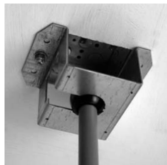
Hang straight bracket and pendant Figure B
